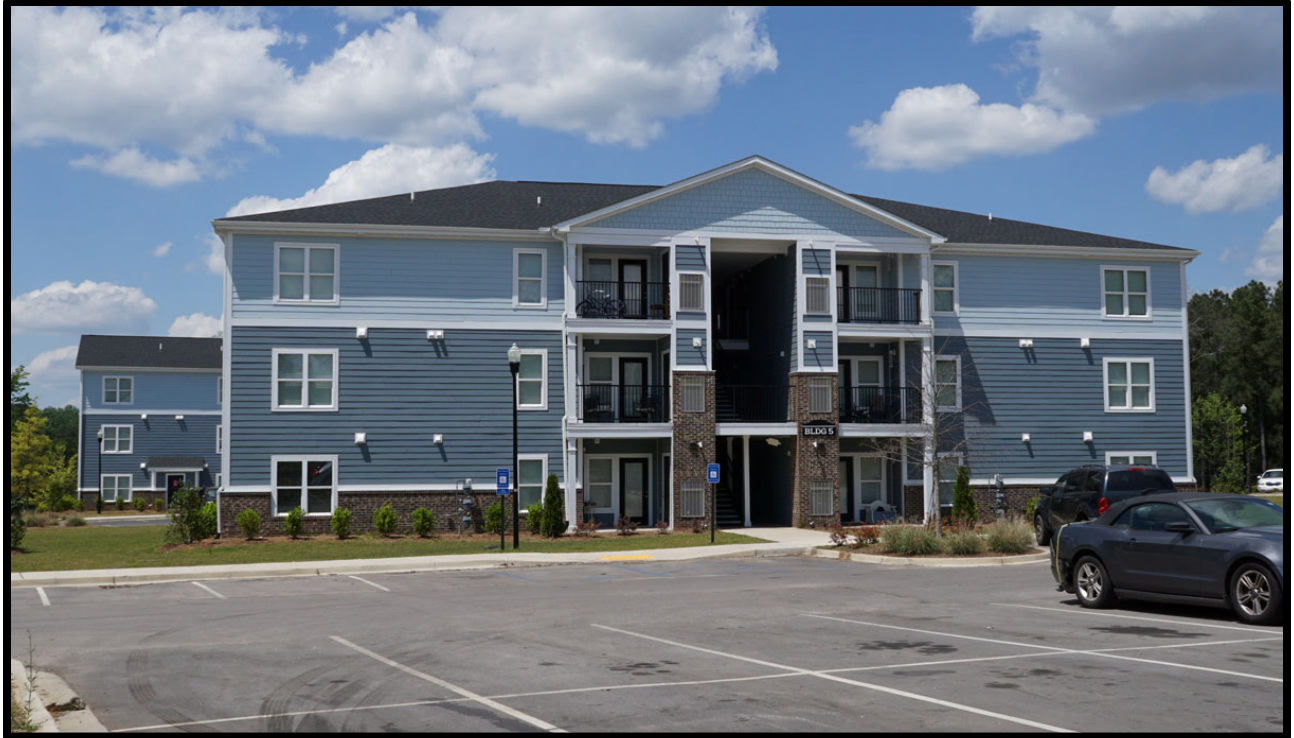
Photo 9—Lorick Place Apartments adjacent to the site (west).
