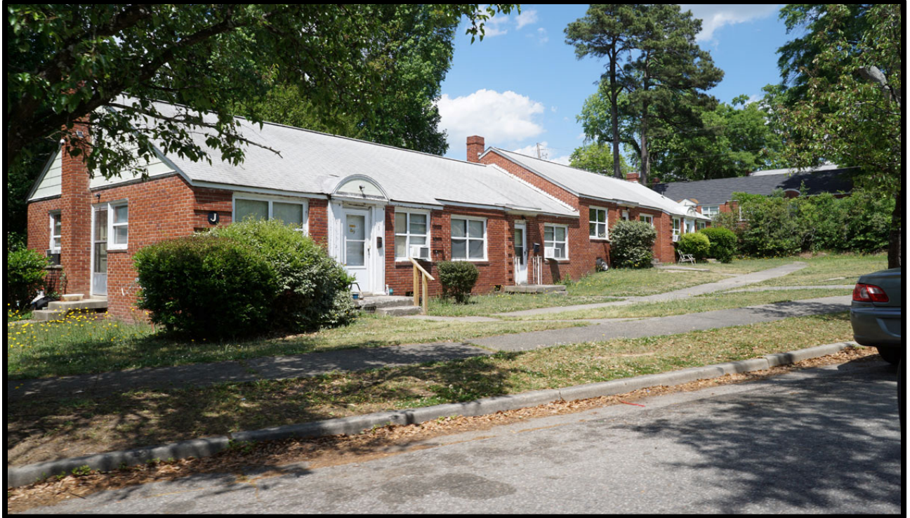
Photo 3—Apartments adjacent to the site on Medical Drive
