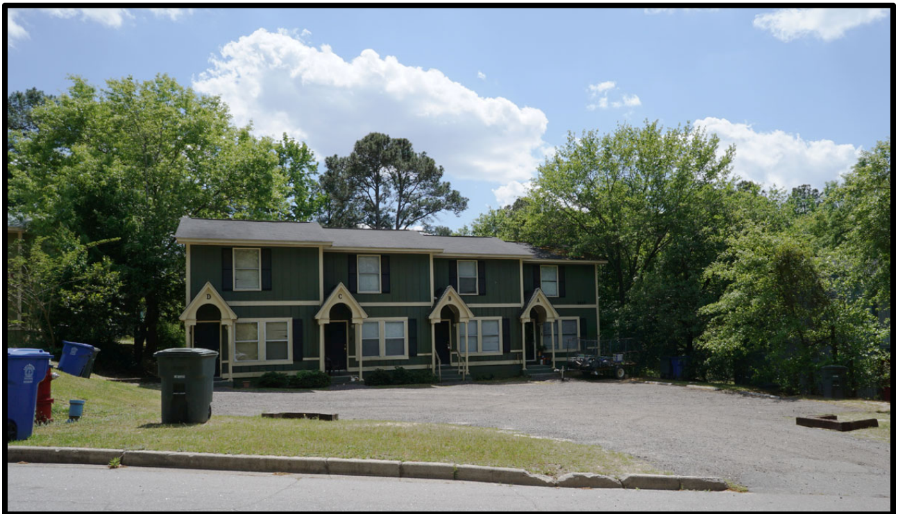
Photo 2—Apartments adjacent to the site on Medical Drive
