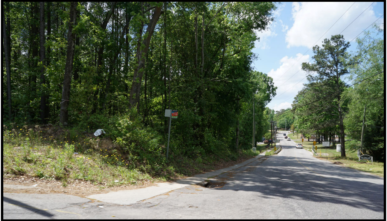
Photo 5—Looking west on Lorick Avenue; the site is on the left. Note the bus stop.
